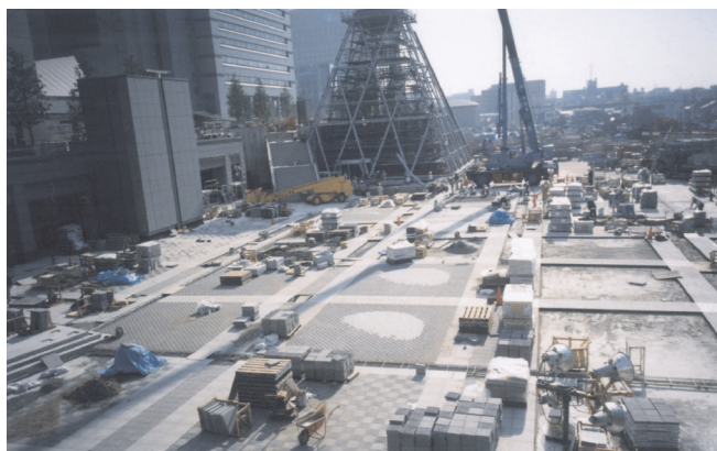
Construction in process
